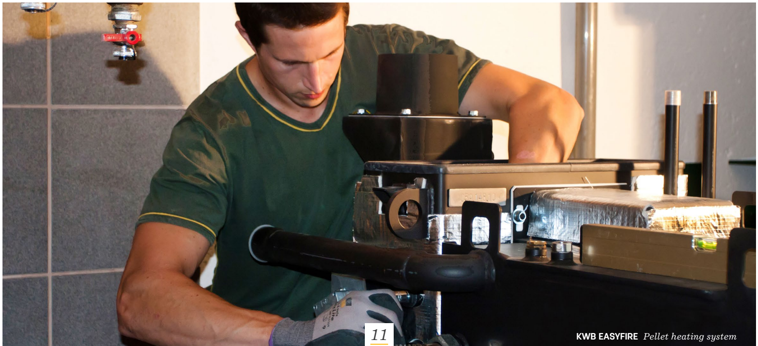
KWB Easyfire – boiler can be dismantled into 2 parts
